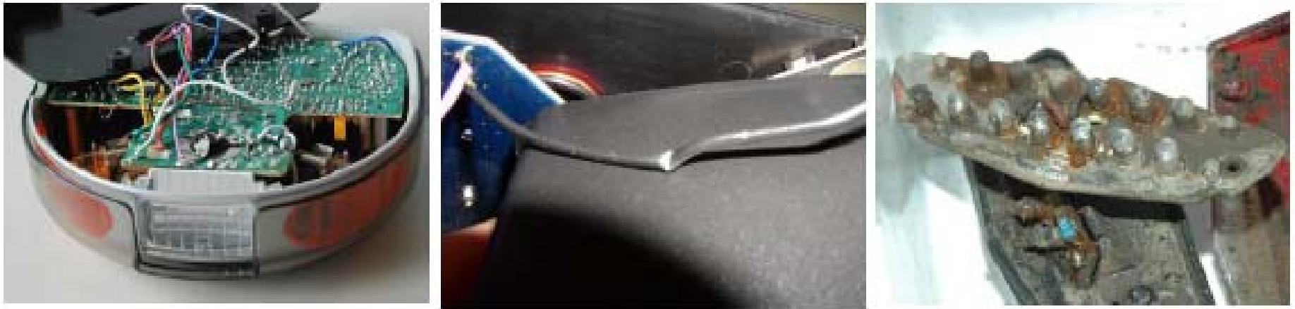
Figure 6-3: Cable spaghetti ( left ), wedged wire ( center ) and heavily corroded components ( right )
